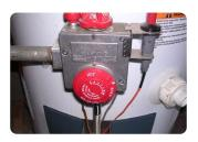
Adjust hot water heater dial between low and medium (~120 degrees F) to prevent accidental scaldings.
